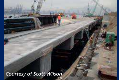
Container Terminal No. 9, Hong Kong
