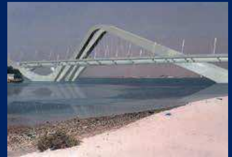
Sheikh Zayed bridge, Abu Dhabi, UAE
